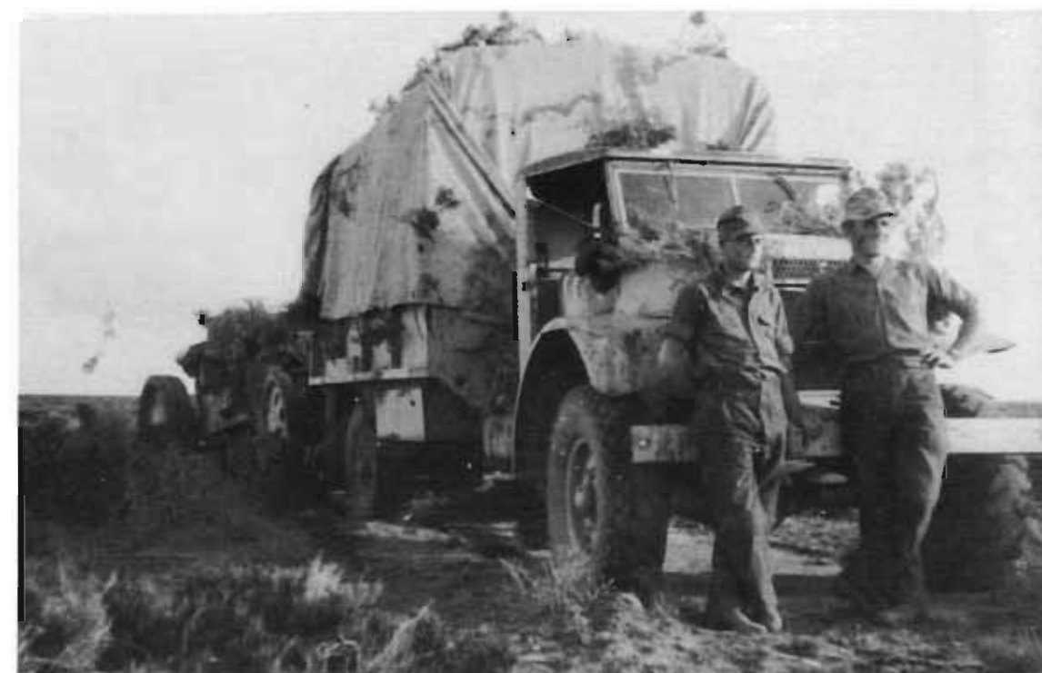
Ford and Chevrolet built 209,000 Canadian 3-ton trucks, which had different motors, gearboxes and rear axles, but most of their other components were interchangeable. The main visible difference was the grille pattern, the Ford's square, the Chevrolet's weblike –as shown here. The C 60 could tow a 15 cm heavy Field Howitzer 18.
