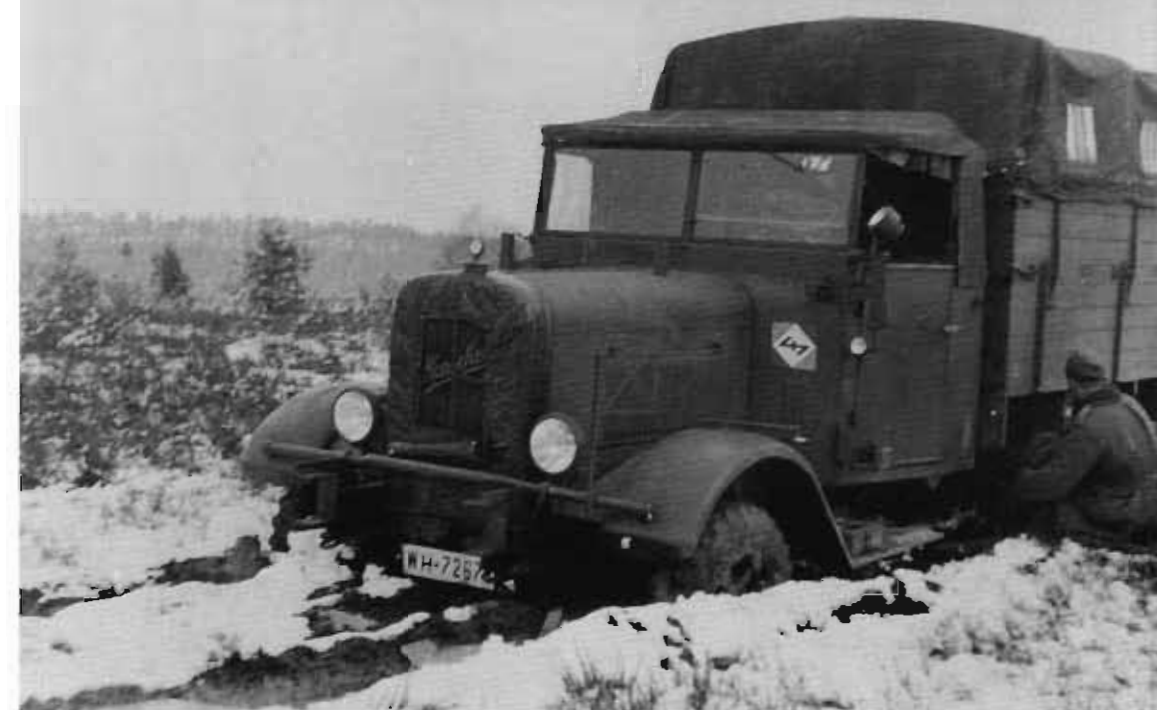
Driving school (off-road) at Grafenwöhr in March 1937. The (prewar) "lying double 7" symbol indicated Engineer Battalion 7 of Rosenheim. The Henschel Type 33 was built with various bumpers, this one the simple tube form of an early series. Note the U-shaped attachments for engineering equipment on the ends of the frame.
