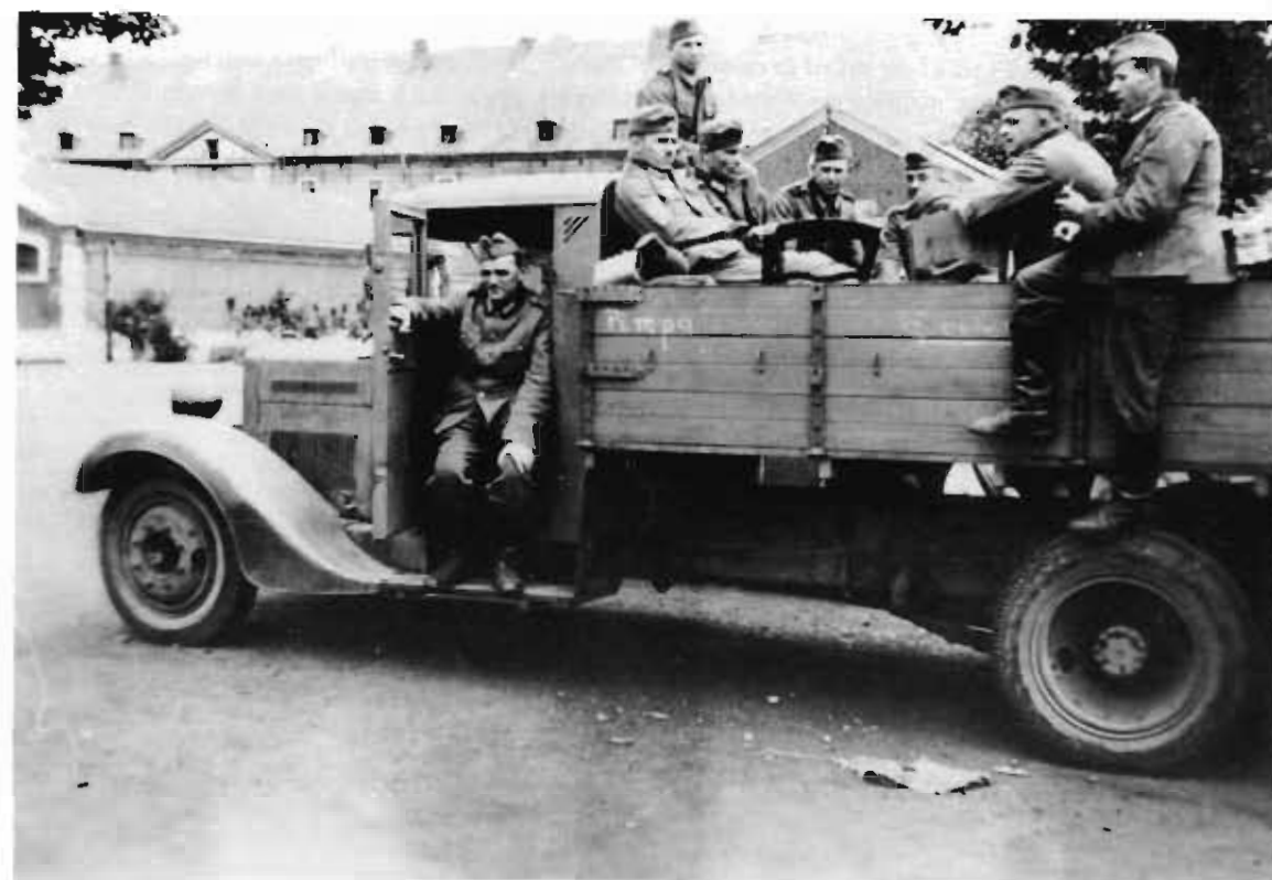
The Polish Polski Fiat 621 L (Fiat license) was built since 1931, with 12,600 built in all. The 4 x 2 vehicle had a load limit of 2.5 to 3 tons and a 50 HP motor. Photos of its use by the Wehrmacht, as here, are comparatively rare.
