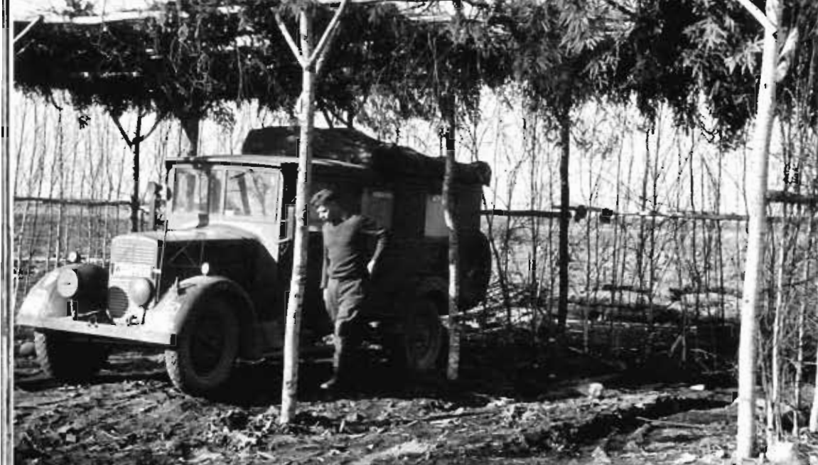
Phänomen Granit 25 H Ambulance (Kfz. 31, WH-12280) with the tactical symbol of an ambulance platoon and the emblem of the 61st Infantry Division. This vehicle had an air-cooled 4-cylinder 2.5-liter gasoline engine that produced 37 HP.
