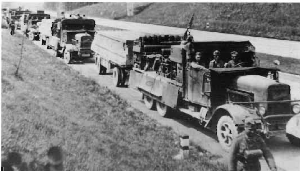
A Bridge Column B on the Autobahn: Henschel Type 33 as Engineer Truck 1 with Pontoon Truck (Pf. 11). The MG 34 gun, carried according to plan, is mounted on turning AA struts. Most trucks used by the grenadier and engineer companies were equipped with a "bottom hole for attaching the mount" in the bed, to be covered by a flap.
