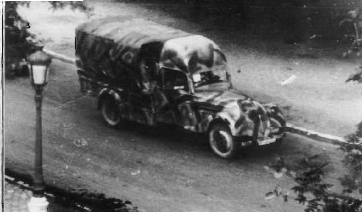
Some 14,000 of the Peugeot DK 5 light truck (1.4 tons, 4 x 2, 45 HP) were built for the Wehrmacht, with either open or closed bodies. The picture shows a Waffen-SS truck at Soignies on 9/3/1944.
