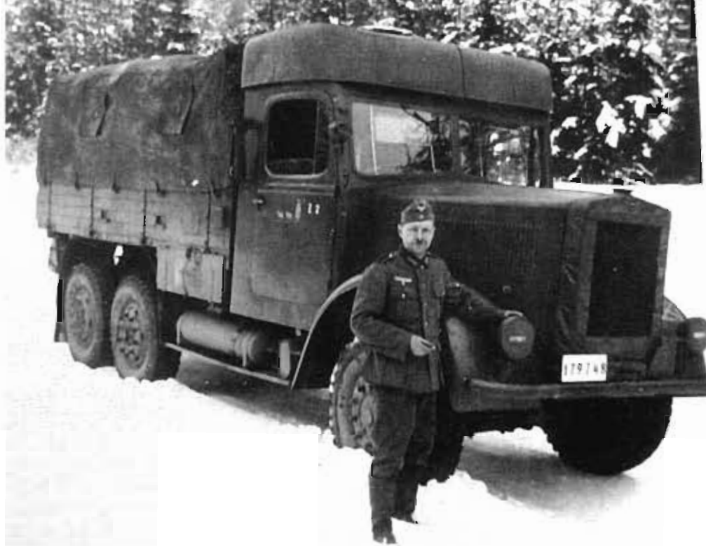
The Czech Skoda H (6 x 4) had a load limit of 4 tons and a 6-cylinder, 8.2-liter gasoline engine with 100 HP. This Skoda (still with Czech registration above) was driven by Georg Birkmeyer in the French campaign as a tool delivery truck of the 212th I.D. (repair-shop company). On the door are "Z 2" and a (blue) shepherd with two sheep, symbol of the company leader, Oberleutnant Schäfer.
