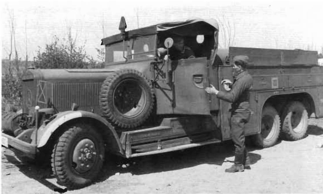
Two views of an "aviation fuel tank truck (Kfz. 384) with chassis of the medium off-road truck (o)", a Mercedes-Benz Type LG 3000 of J.G. 2, in northern France in 1942. Note the location of the exhaust pipe under the front bumper, customary for tank trucks, the slit cover of the main headlight, and the tires with the fairly uncommon "Wehrmacht tread." The tank had a capacity of 3500 liters of fuel.
