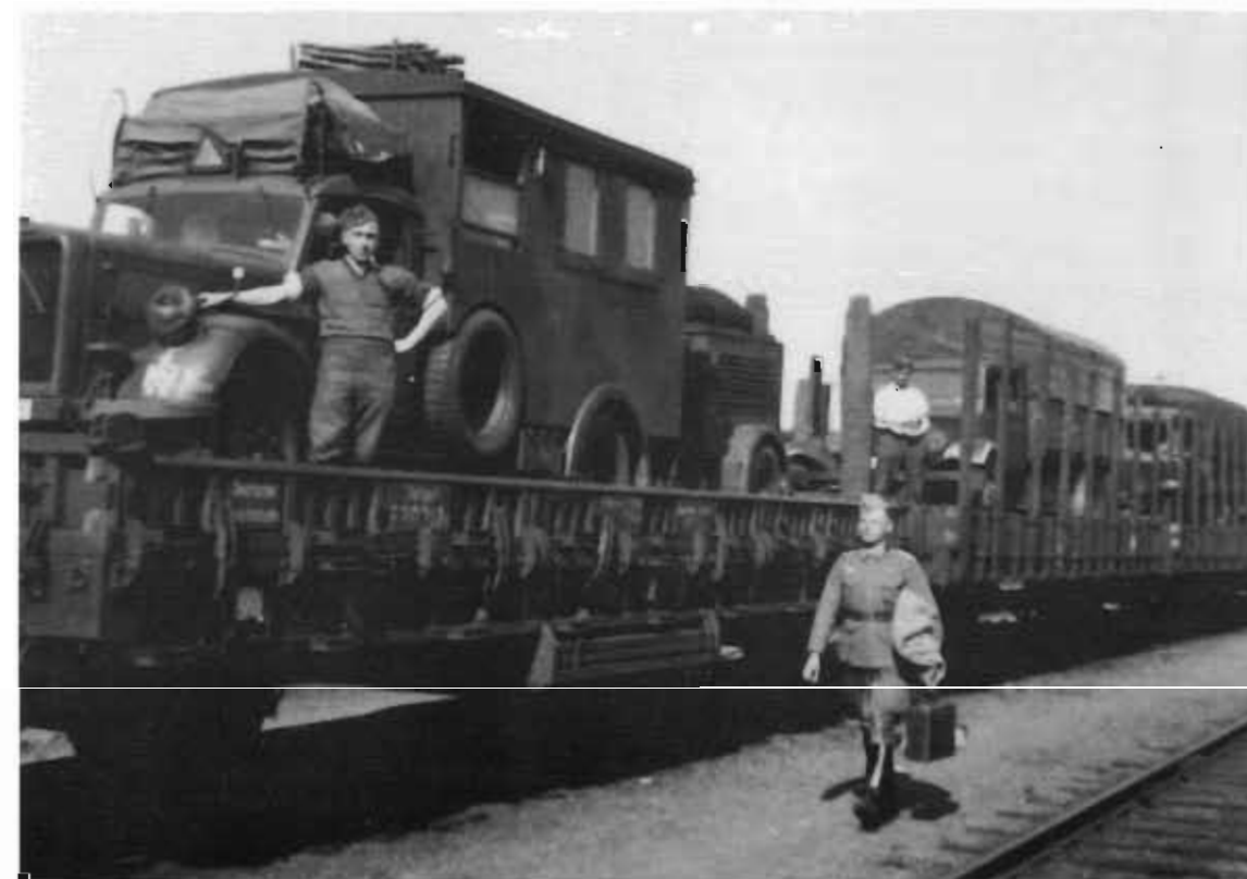
The 3-ton Borgward with box body and rigid cab was relatively rare. This is a vehicle of Panzer Observation Battery 322 (Later Pz.B.B. 90), which was subordinate to the 10th Panzer Division, equipped as Evaluation Vehicle Kfz. 62 with Special Trailer 23 (battery-charging device).
