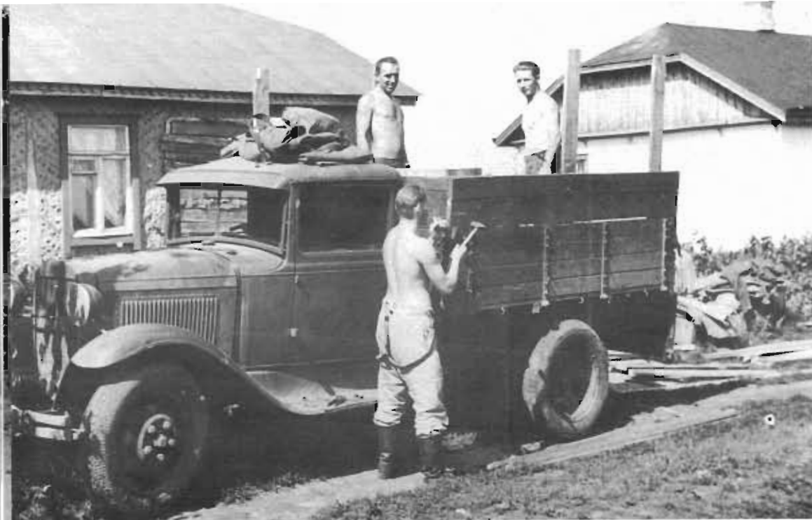
The Russian motor vehicle industry built its trucks almost exclusively under American Ford and Autocar licenses of the early thirties. The vehicles thus were technically obsolete but sturdy and easy to repair. In this picture, a GAZ-AA (1.5 tons, 4 x 2, 40 HP) of Engineer Battalion 260 is acquiring a closed body for field use.
