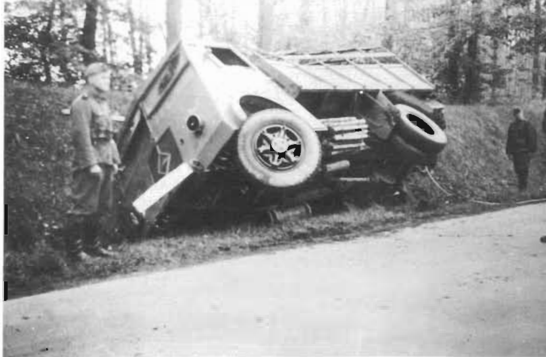
This truck (SS-109625) of the 5th SS Panzer Regiment "Viking" was wrecked during a transfer from Wildflecken to Sennelager in May of 1942. It is a Renault AHN (3.5 tons, 4 x 2, 75 HP) that was built in large numbers for the Wehrmacht.
