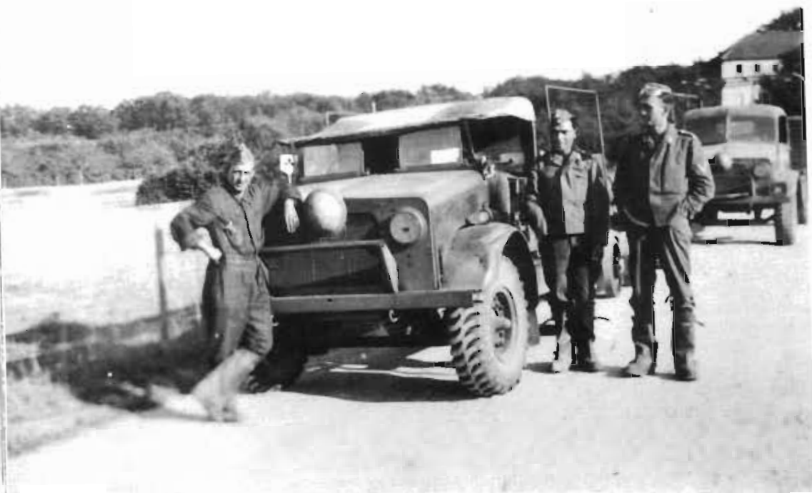
During the war, Vauxhall Motors produced the impressive quantity of 66,000 Bedford MWD trucks (0.8 tons, 4 x 2, 72 HP). This picture shows a captured truck of the Luftwaffe, with a 3-ton Bedford OYD in the background.
